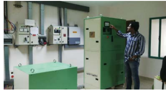
Fig. 2.3. Photograph of Solar PCU developed by CDA
